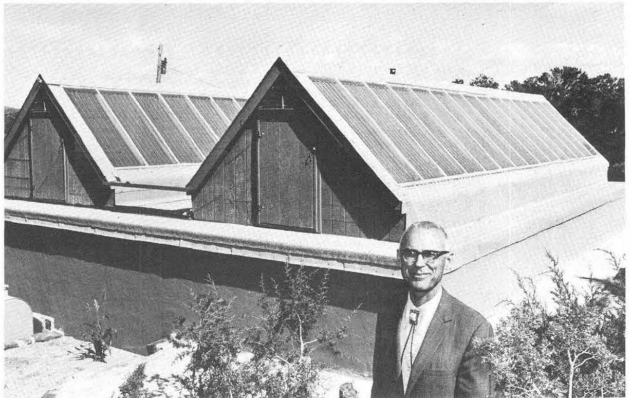
DALE HASKINS (4714) built these solar collector structures on top of his garage some 30 ft. from his house. Solar heated hot water circulates into a thousand gallon heat storage tank in the garage and then into a baseboard radiation heating system in the house. The solar system provides 85 percent of his space heating needs and 100 percent of the hot water.
